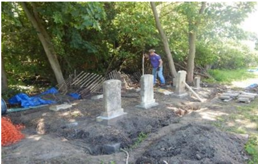
Restoration Work in Progress
